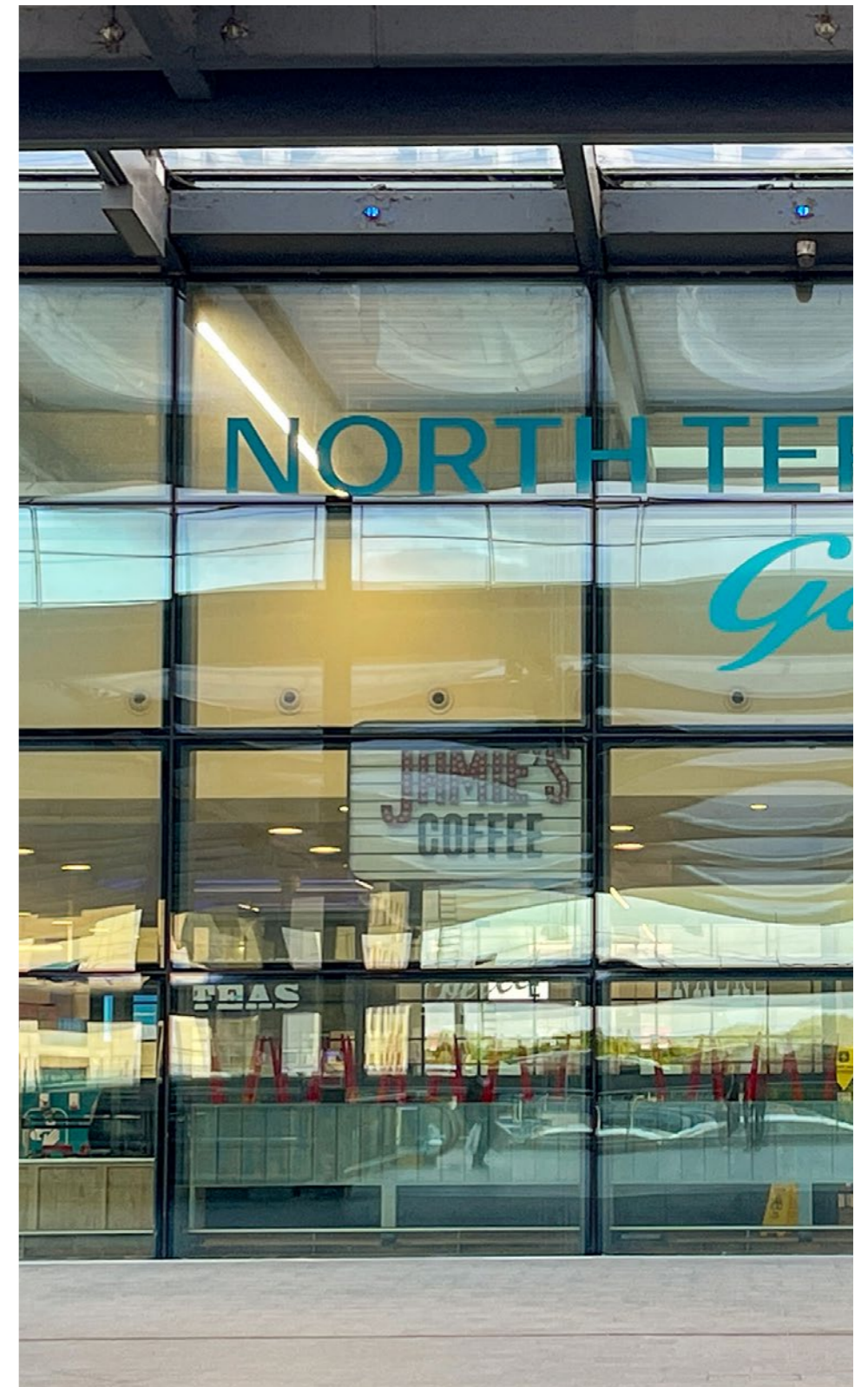
Figure 16. North Terminal forecourt facade
