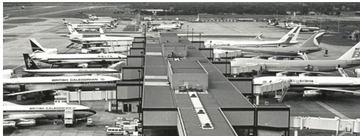
Figure 11. Gatwick Airport 1970s
